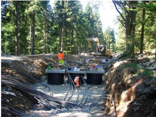
200 km cables for power supply, data transmission and backup communication lead to each seismometer vault in a star-shaped layout. All cables are merged in the main cable duct to the central facility.
