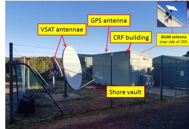
As more frequent and strong lightning strikes were observed in the vicinity of the HA01 CRF, the CRF will be upgraded with a lightning protection system in-line with the CTBTO best practices. The figure above shows the HA01 CRF.
